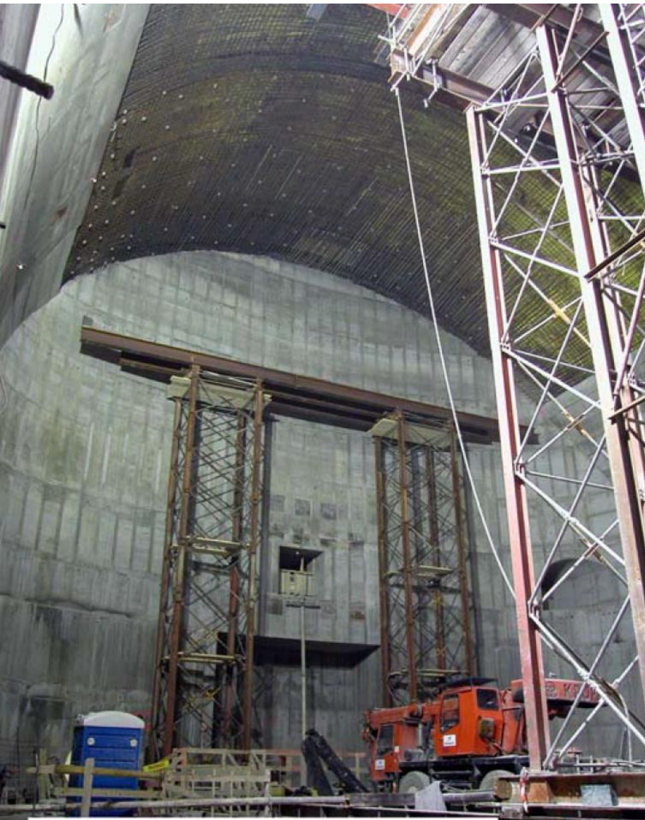
LHC Point 5 - UXC55 Point 4 End Crown Falsework - 29-03-2004 - CERN TS/CE
