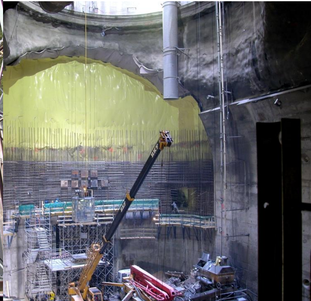
Point 6 headwall - 20-06-2003 - CERN ST/CE
